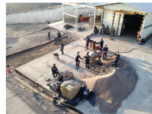
Crews installing concrete near the surface maintenance shop at Platosa
