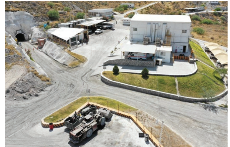
Aerial view of the portal, shops and administration facilities at Platosa
